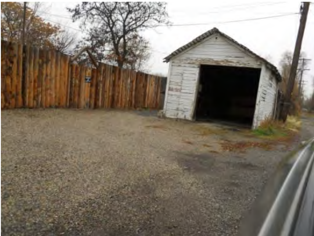
View of garage from 562 East Stratford
